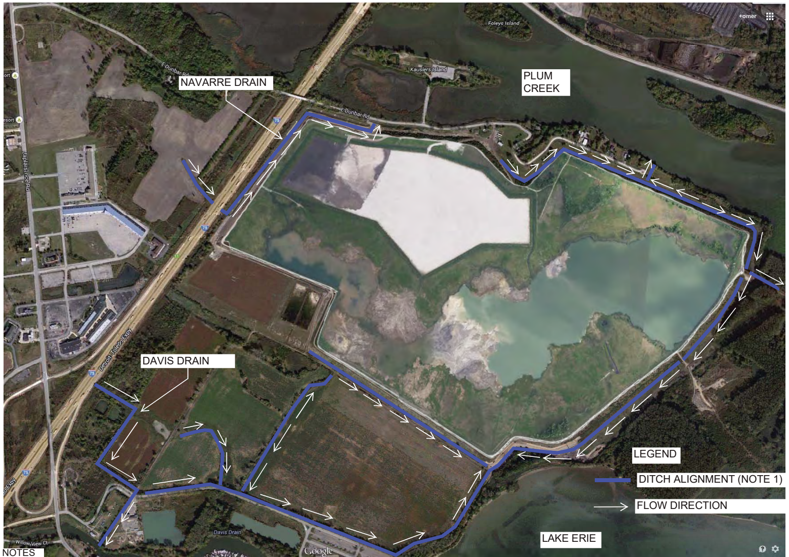
FIGURE 5. APPROXIMATE ALIGNMENT OF EXISTING DITCHES AND FLOW DIRECTIONS IN THE FLY ASH BASIN AREA
